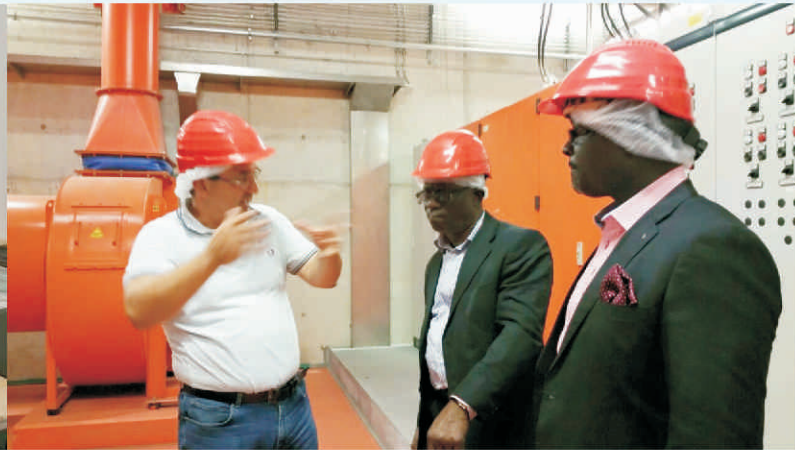
At Borzano Power Plant, Italy
